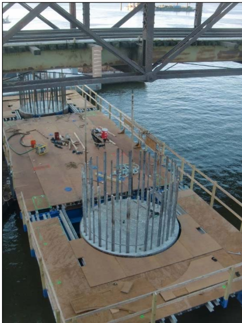
Figure 3 - Drilled Shafts installed with oscillator outside of existing bridge footprint
