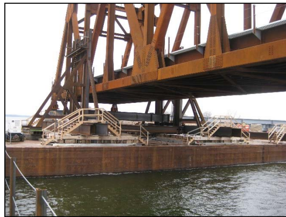
Figure 9 - Sandbox support method on barges
