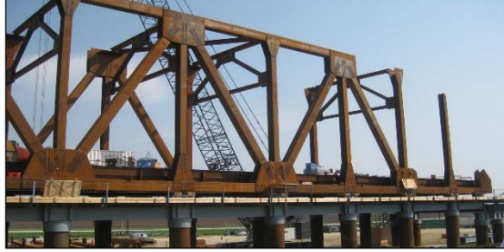
Figure 5 - Work platform used for truss erection
