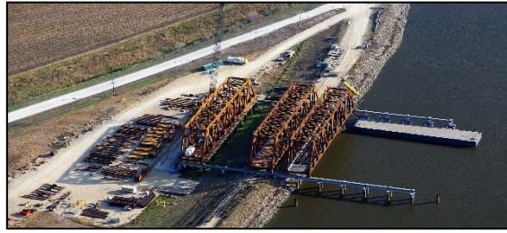
Figure 2 - Approach Span Trusses 2-6 erected 13-miles downstream
