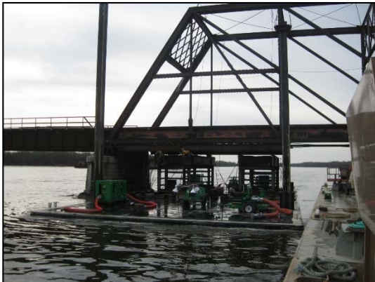
Figure 10 - Barge under existing truss prior to track closure
