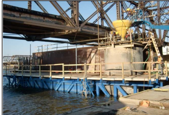
Figure 4 - New pier cap installed with floating formwork
