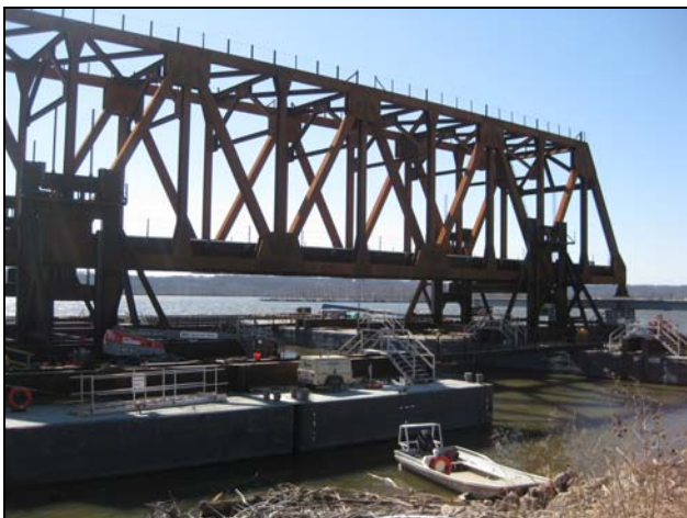
Figure 9 – Approach span truss loaded onto float-in barge jacking towers
