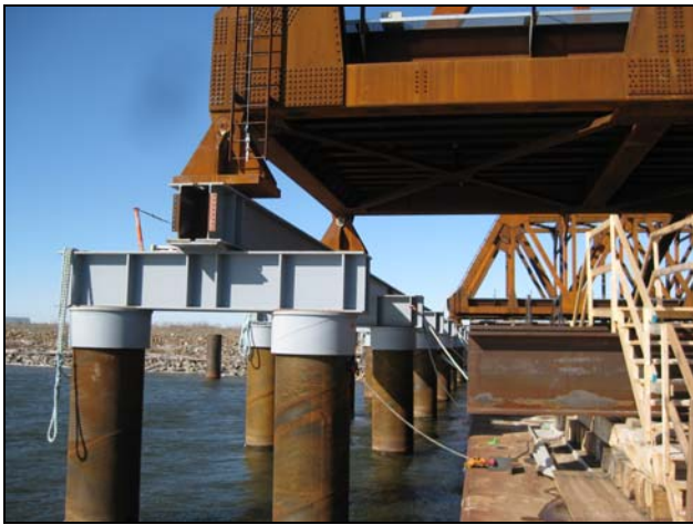
Figure 8 – Typical track beam system pile bent
