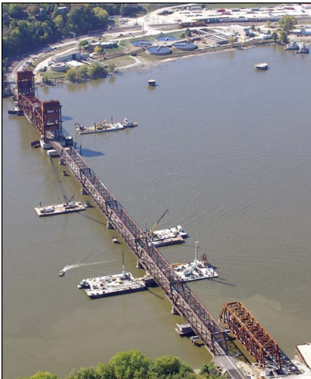
Figure 2 – Approach span truss # 1 erected at job site
