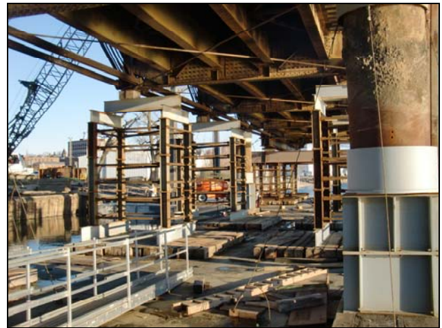
Figure 21 – View of third barge and additional tower support provided during demolition
