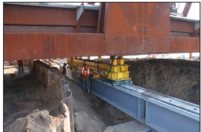
Figure 7 – Push/Pull frame and reaction sled shown at approach span truss # 1
