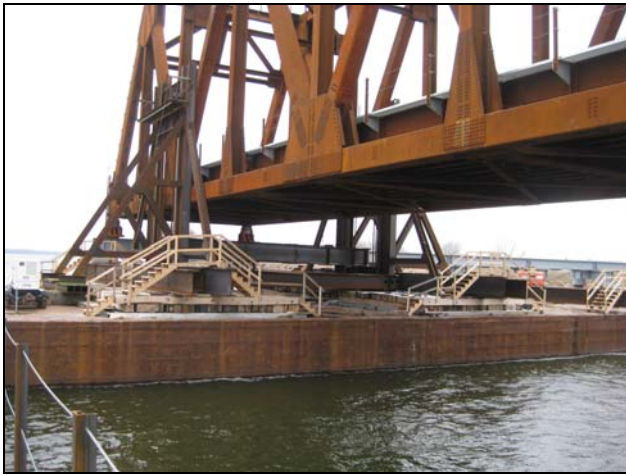
Figure 12 – Sandboxes support method on barges
