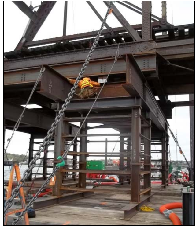
Figure 17 – Bottom chord and W24 underslung beam used to deliver load around vertical hanger designed for tension
