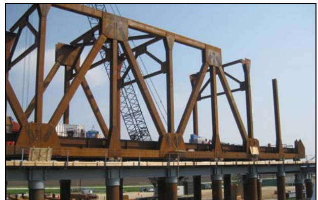
Figure 4 – Work platform used for truss erection
