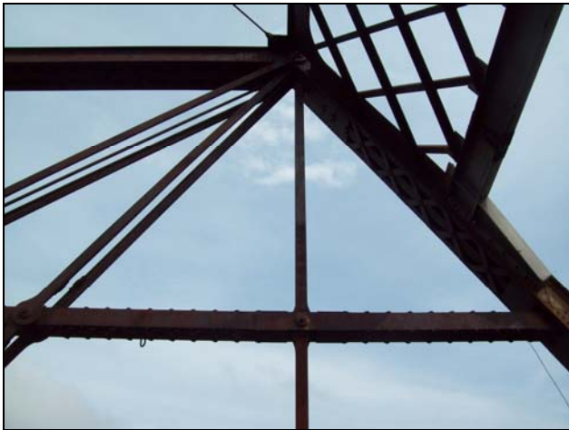
Figure 16 – Vertical hanger at panel point 1
