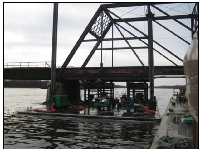
Figure 18 – Barge aligned with existing truss in preparation for track closure
