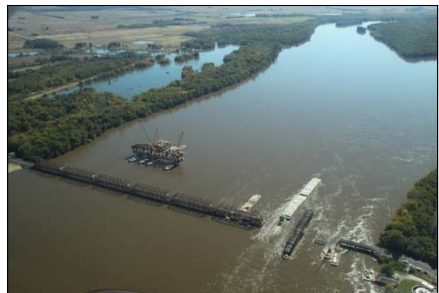
Figure 1 – Existing 120 year old bridge structure with 360-foot Swing Span
