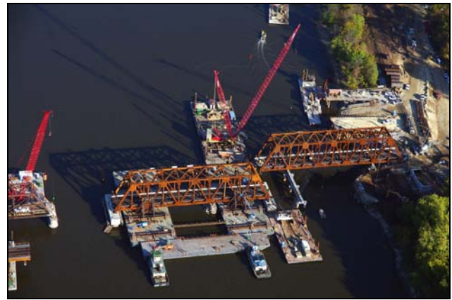
Figure 13 – Tugs positioning truss near final bridge alignment
