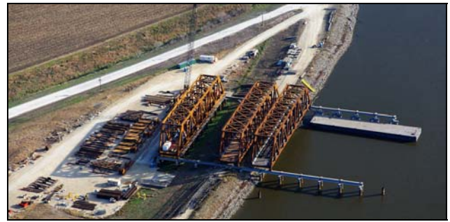
Figure 3 – Approach span trusses 2-6 erected on track system at Green Bay location
