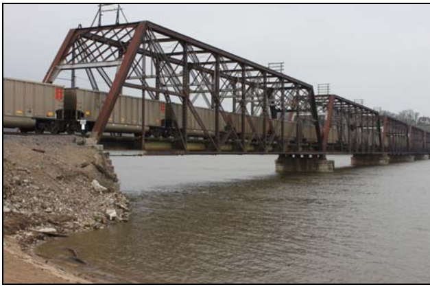
Figure 15 – Existing approach span truss
