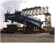
An existing 80-year-old rolling bascule bridge spanning the Maumee River was renovated by the City of Toledo, Ohio. One component of this renovation project was the removal and disassembling off-site of the four existing bascule leaves, and replacing them with four new bascule leaves pre-assembled off-site.
