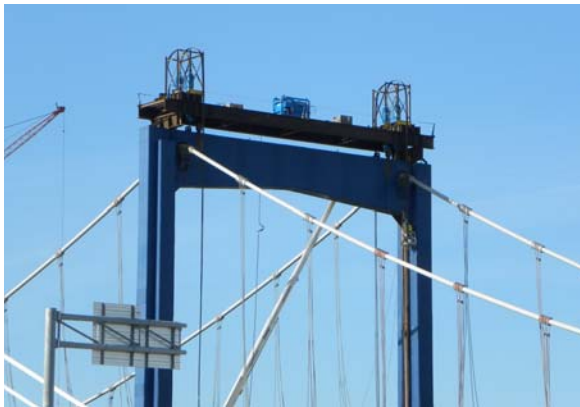
Figure 11 – Strand Jacks for Cable Lowering
