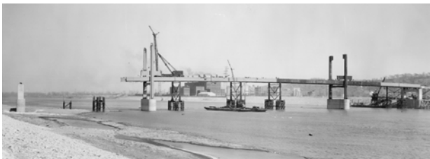
Figure 3 – Stiffening Girder Erection
