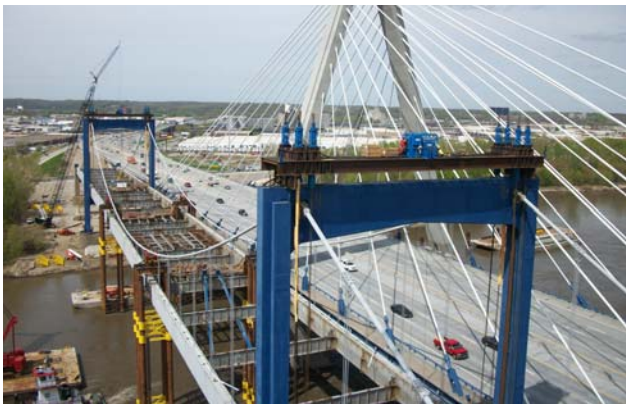
Figure 9 – Strand Jack System
