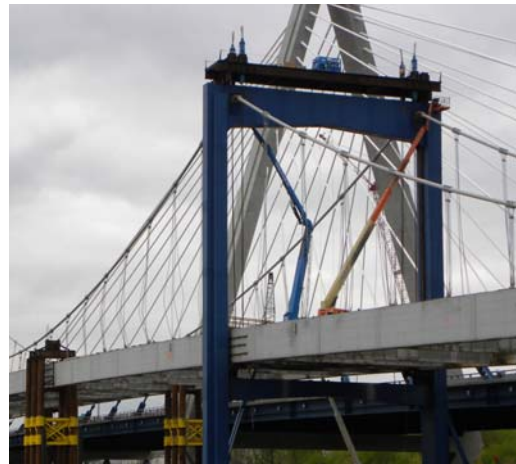
Figure 10 – Suspender Cables after lifting
