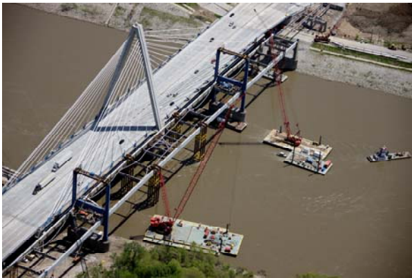
Figure 1 – Paseo Bridge during demolition
