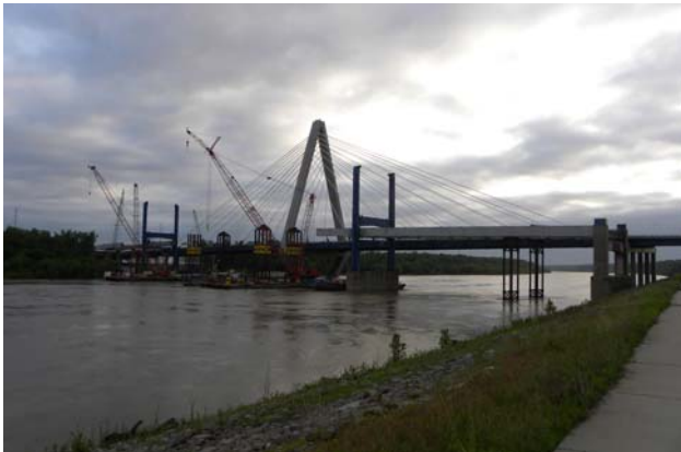
Figure 15 – Stiffening Girder Removal
