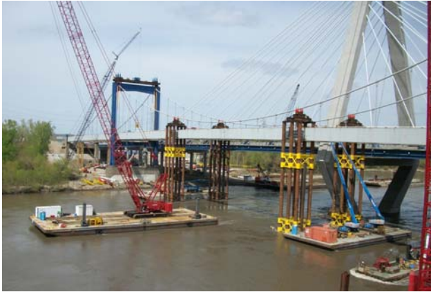
Figure 8 – Falsework Towers
