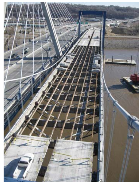
Figure 7 – Slab Removal
