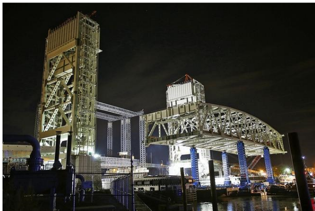
Figure 22 - Truss at Project Site Waiting on Tide
