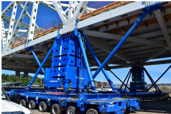
Figure 11 - SPMT & Lifting Towers @ L4
