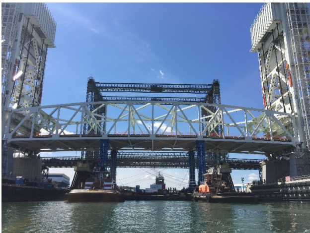
Figure 27 - Barge ready to be pulled from channel
