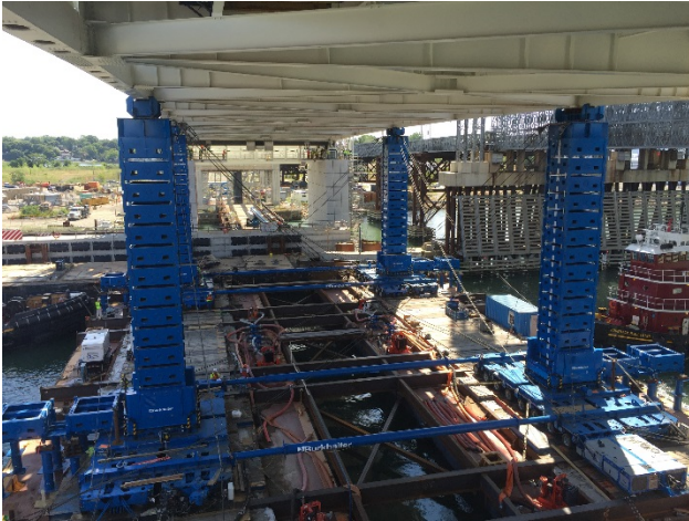
Figure 24 - Truss in Final Position waiting on tide
