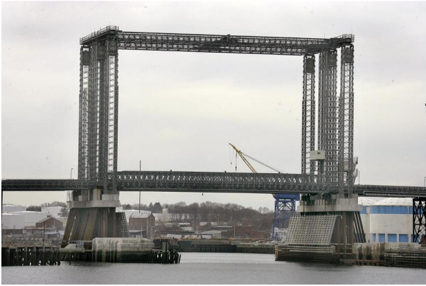
Figure 3 - Current ACROW Lift-Bridge
