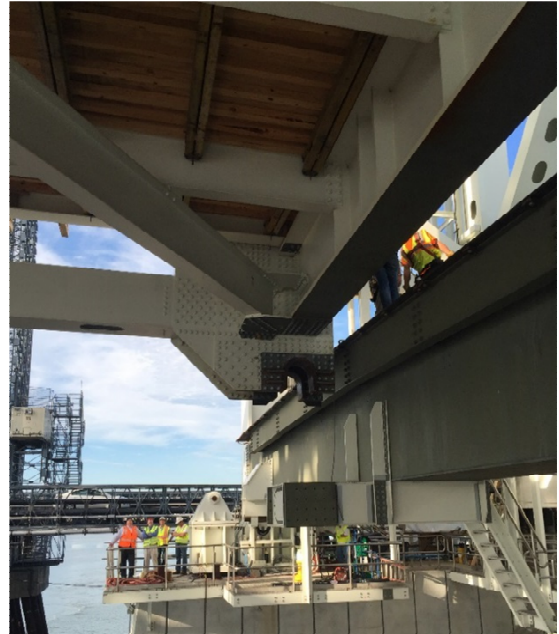
Figure 23 - 3" Working clearance each end of truss
