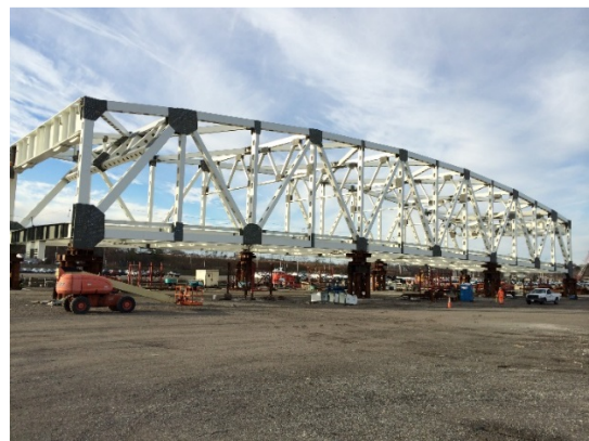
Figure 10 - Erected Truss on Falsework Towers
