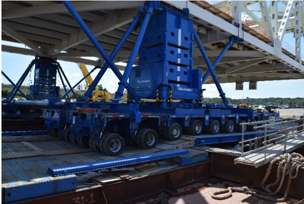
Figure 14 - SPMT's traveling over Ramps onto Barge
