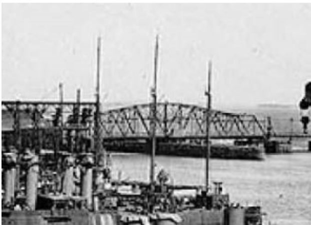
Figure 1 - Original 1902 Swing Span
