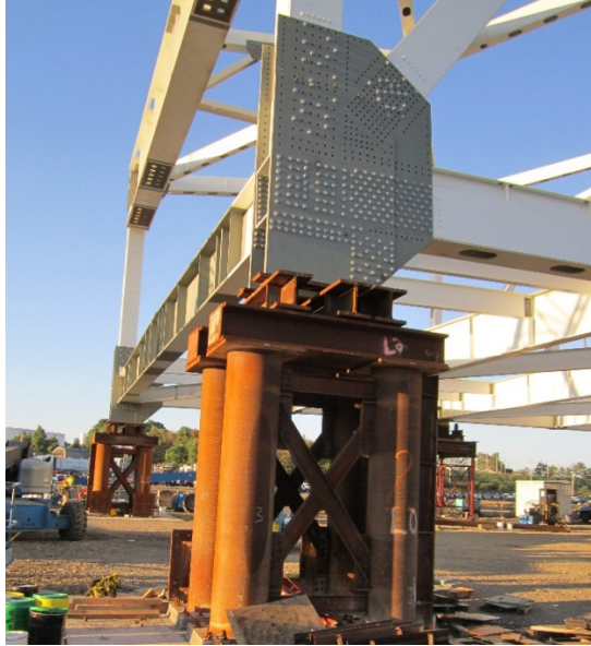
Figure 7 - Temporary Heavy-Duty Erection Tower (shown at L0)
