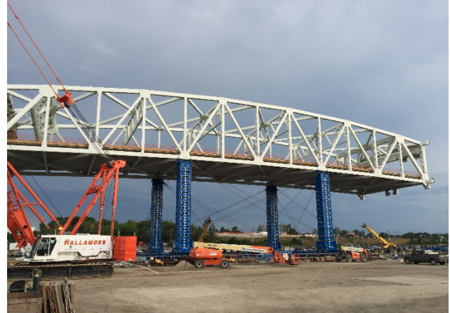
Figure 19 - Truss lashed to truss after lifting
