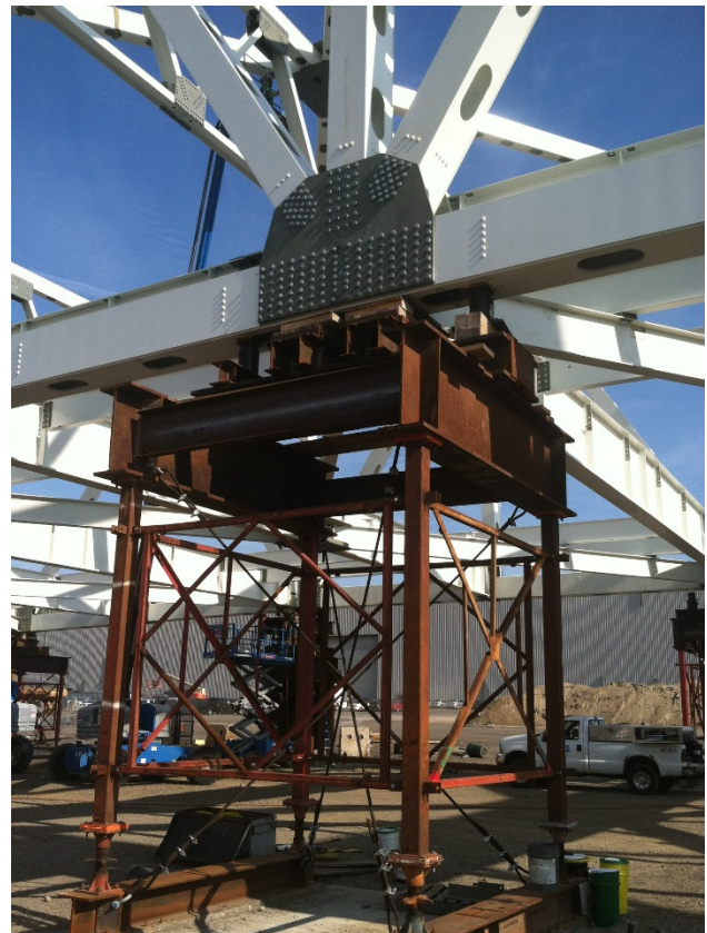
Figure 6 - Temporary Lite-Duty Erection Tower
