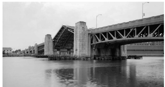
Figure 2 - 1936 Replacement Bascule Span
