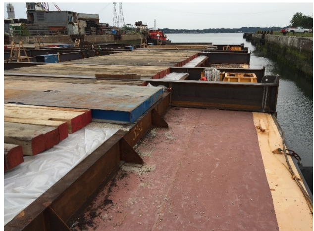
Figure 17 - Sandbox & Mats Distribute Transport Loads
