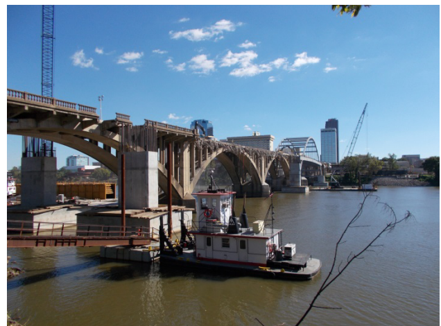
Figure 3 - New Bent Construction
