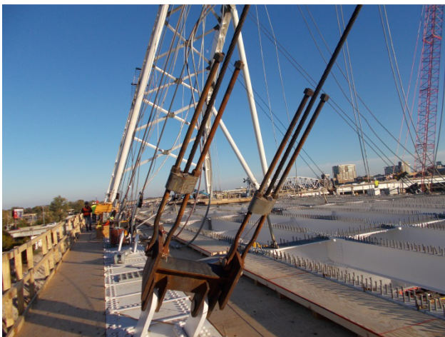
Figure 14 – Temporary Hanger Bracket & Adjustable Lower Socket
