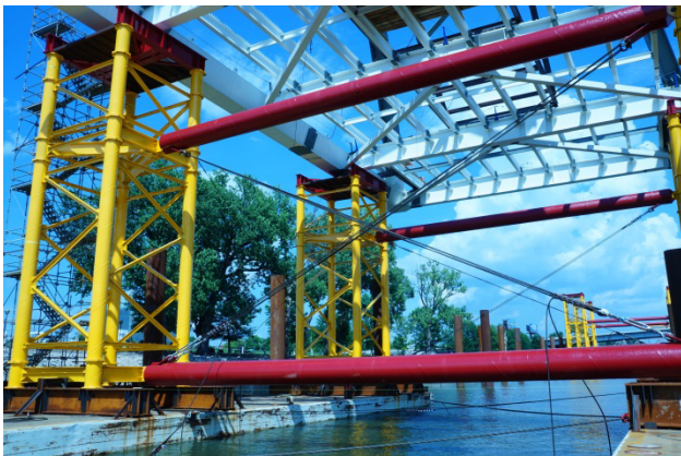
Figure 7 - Falsework Grillage & Bracing System
