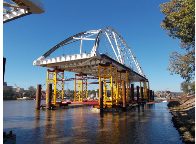
Figure 2 - Accelerated Bridge Construction
