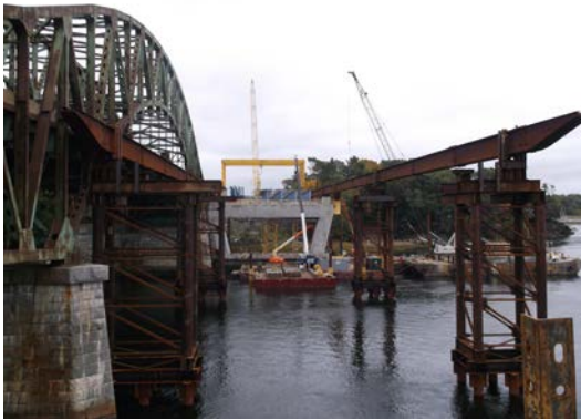
Figure 12 – Pipe Column Falsework Towers
