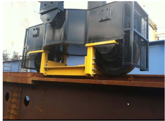
Figure 8 – Overhead Crane Rail & Splice Interface
