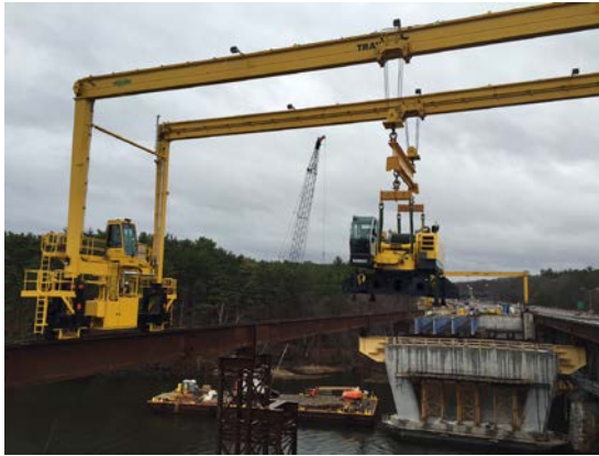
Figure 15 – 200-ton Crane Assembly
