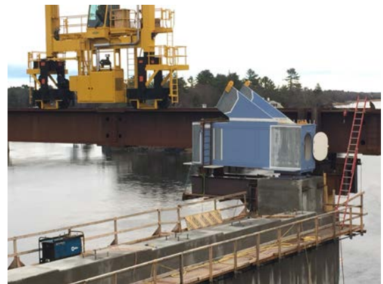
Figure 14 – Arch Floor System Erection
