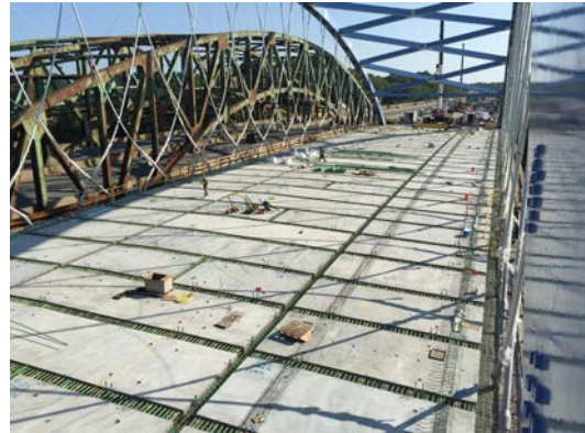
Figure 17 – Precast Deck & Cable Hangers Installed
