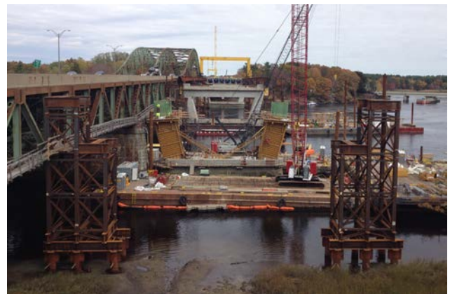
Figure 11 – W-Column Falsework Towers
