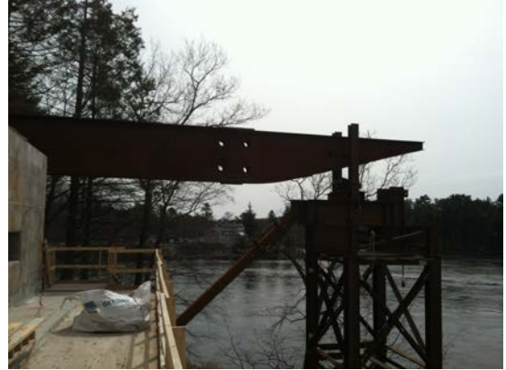
Figure 5 – Launch Girder Nose
