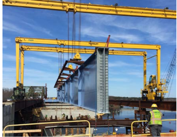
Figure 2 – Overhead Cranes Deliver Steel
