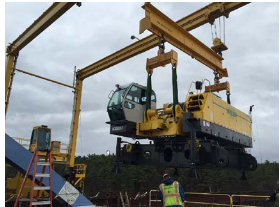
Figure 3 – Overhead Cranes Deliver Crane
