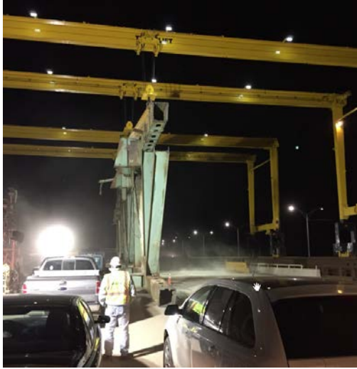
Figure 4 – Overhead Cranes Used for Demolition
