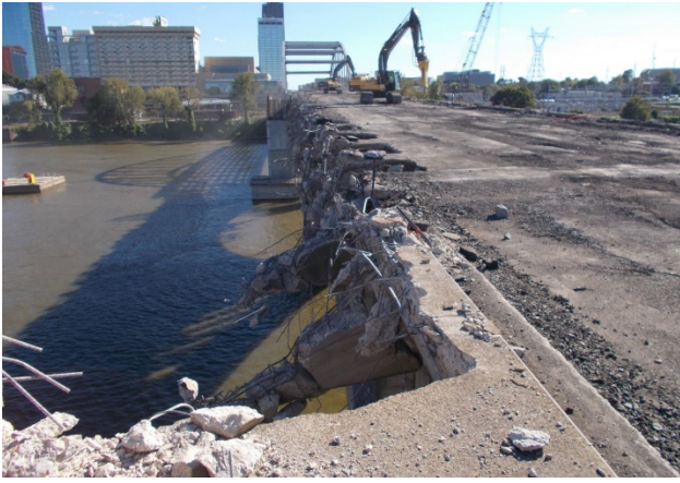
Figure 15 – Deck Overhang Removed
