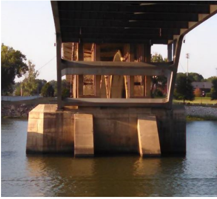
Figure 9 – Counterweight Added to Pier 2
