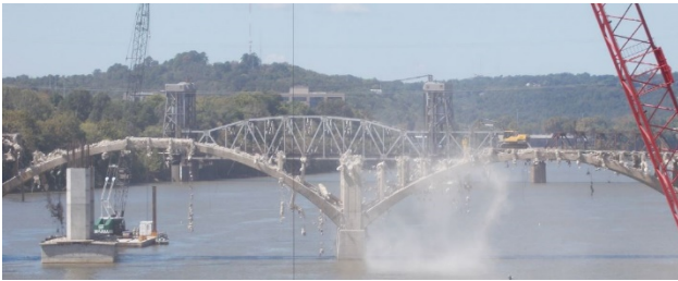
Figure 16 – Excavator Deck Removal
