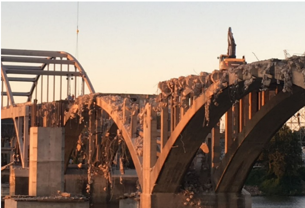
Figure 17 – Excavator Deck Removal
