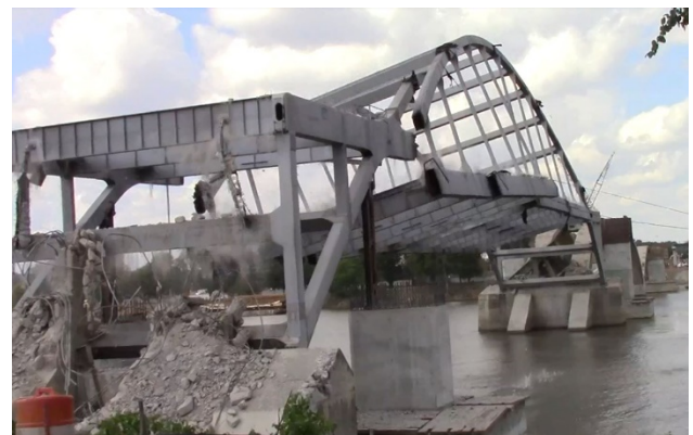
Figure 22 –Steel Arch Span
