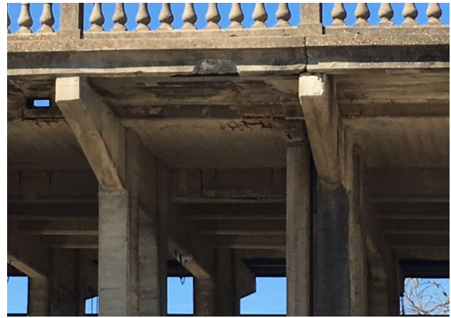
Figure 6 – As-Built Spandrel Columns
