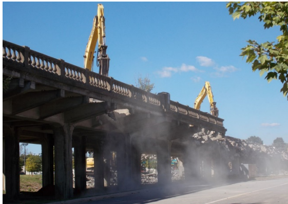
Figure 12 – Multiple Excavators on Deck
