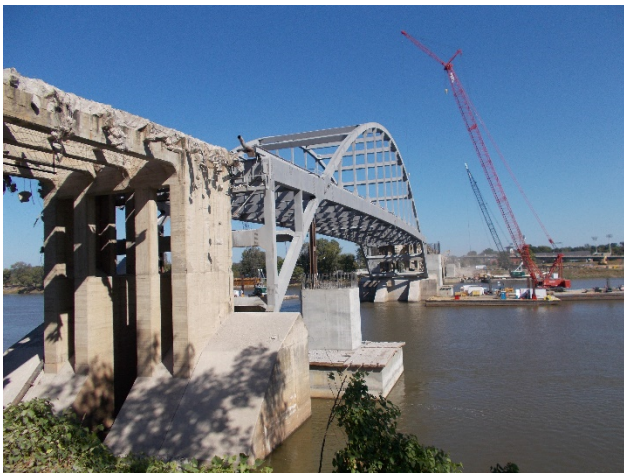
Figure 20 – Arch Support System
