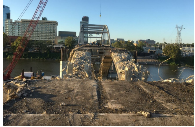
Figure 18 – Edge of Deck Removal
