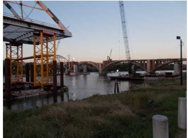
Figure 19 – New Bridge Supported on Falsework with Demolished Bridge in Background
