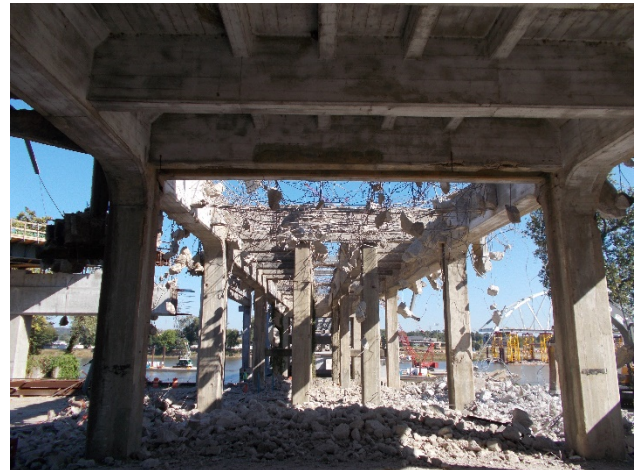
Figure 14 – Deck Removed in Approach Spans
