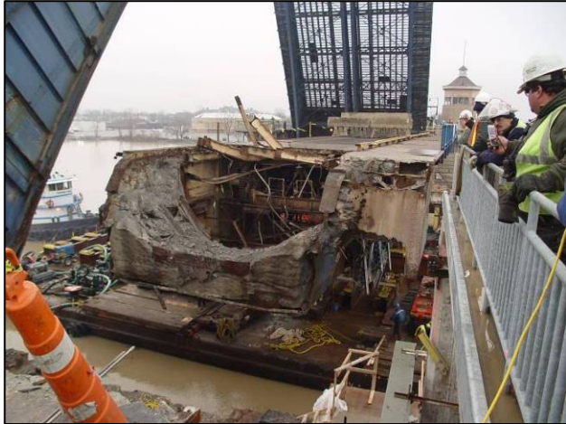
Figure 9 – 15% of the counterweight remained
