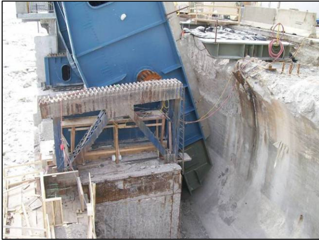
Figure 25 – Bridge opened during machinery tests
