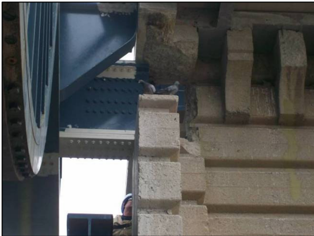
Figure 22 – Final fit up of spans
