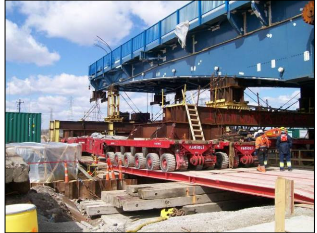
Figure 19 – SPMT's roll "nose" first onto barge
