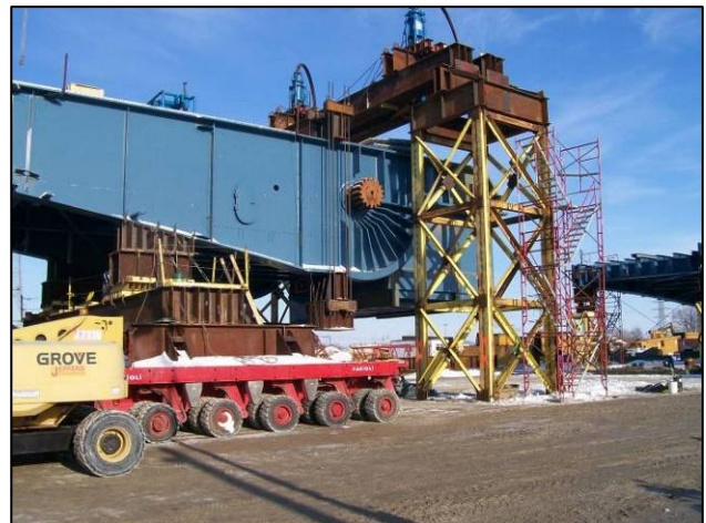
Figure 16 – SPMT's under back gantry
