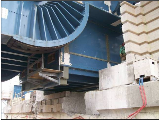
Figure 21 – Initial fit up of spans
