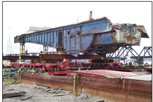
Figure 11 – SPMT's backing onto ramps
