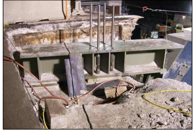
Figure 23 – Installation of live load anchors
