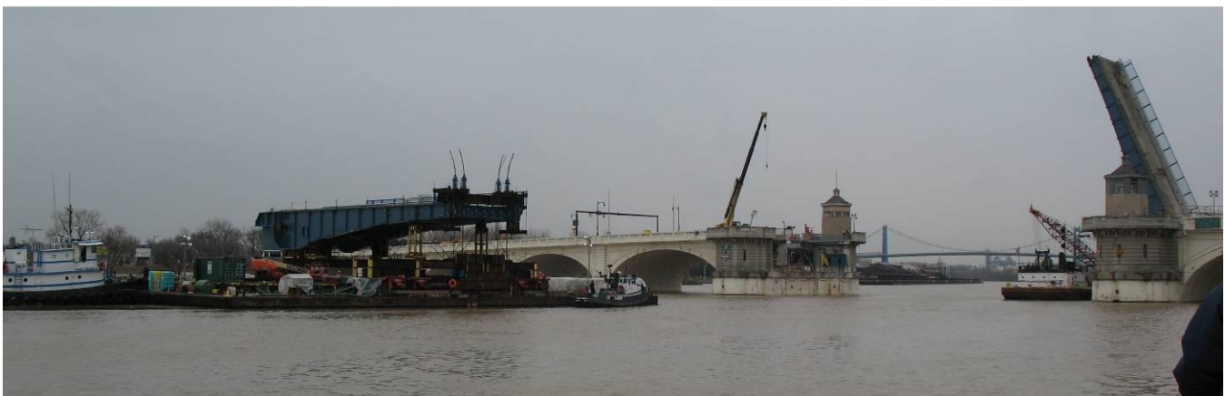
Site Photo – Second New Bascule Leaf is Floated into Position
