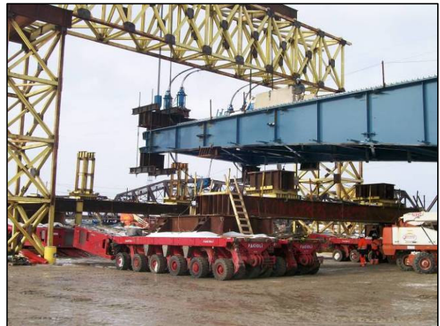
Figure 15 – SPMT's under front gantry truss
