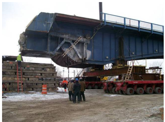
Figure 12 – SPMT's backing into mat cribbing
