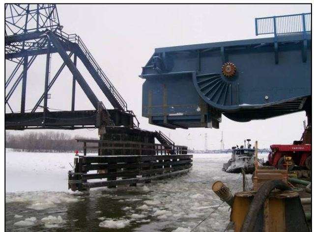
Figure 20 – Tight clearances at existing RR bridge.
