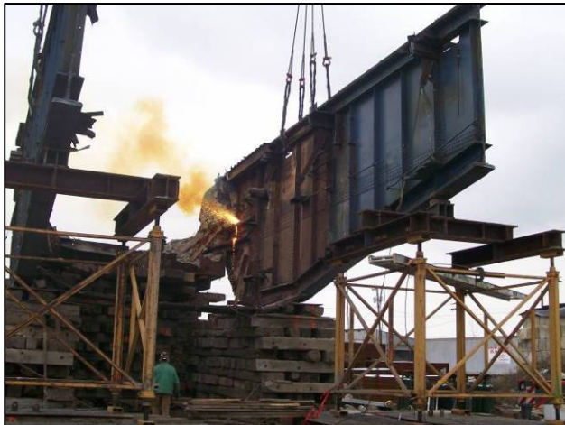
Figure 14 – Surgical type cutting using lances
