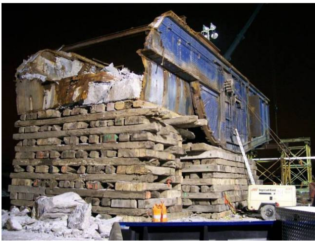
Figure 13 – Timber mat cribbing under steel girders
