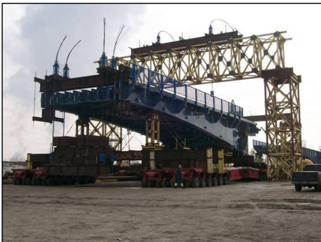
Figure 18 – SPMT's move out from under gantries
