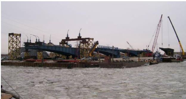
Figure 1 – Steel Erection in Staging Yard
