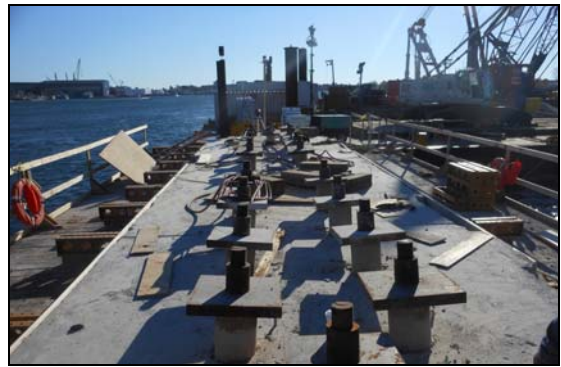
Figure 15 – Micropiles installed in existing foundations
