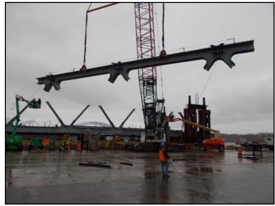
Figure 18 – Top chord segment installation
