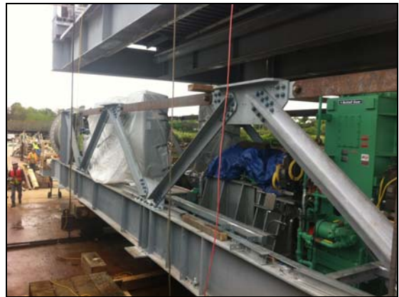
Figure 21 – Machine Room Truss “Temporary” Top Chord utilized during machine room lift
