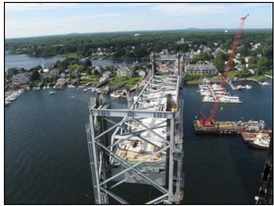
Figure 33 – Adjustments to lift tower continued after lift span balanced and installed
