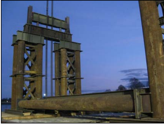
Figure 10 – Falsework Tower System for float-out of Existing Lift Span Truss
