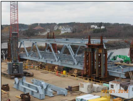
Figure 17 – New Fixed Span Truss partially erected on Cape Cod Barge
