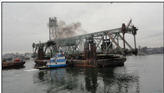
Figure 8 – Lift Span removed and supported on barge
