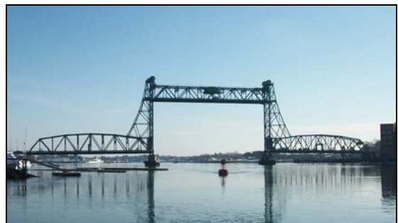
Figure 2 – Bridge still able to perform daily lift activities
