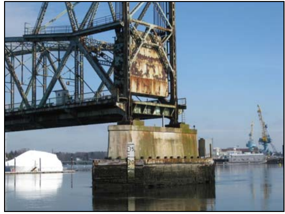
Figure 9 – 900 kip Concrete CTWT prior to demolition
