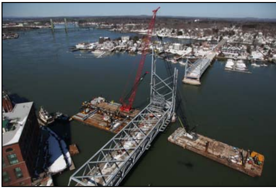
Figure 26 – Lift tower construction of South Fixed Span
