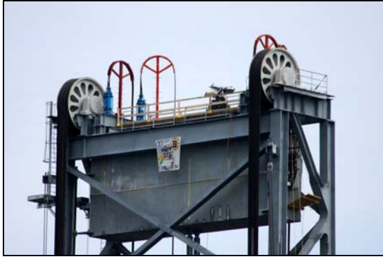
Figure 31 – CTWT in final lifted position, supported by strand jacks
