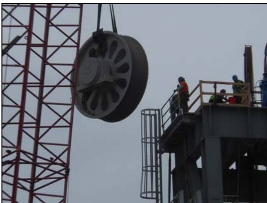
Figure 28 – Installation of 11’-2” Diameter Lift Tower Sheave
