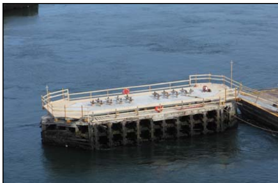
Figure 14 – Existing Pier after span float-outs, strengthened for reuse with new bridge
