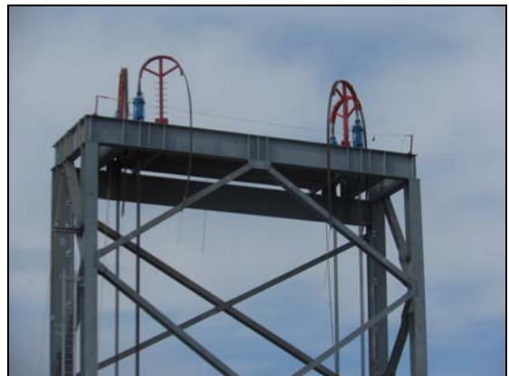
Figure 30 – Strand Jacks Supported by upper lift tower framing
