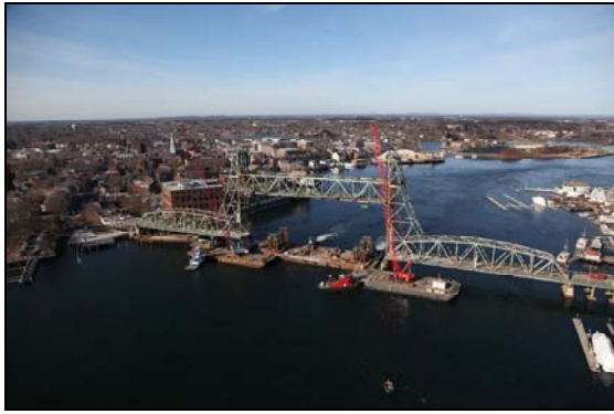
Figure 6 – Original Bridge just prior to demolition
