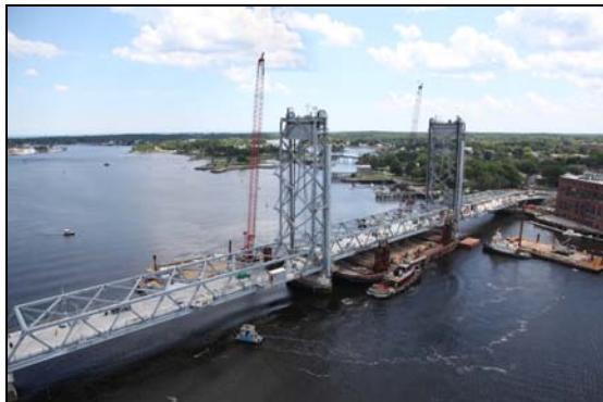
Figure 32 – New Lift Span installed prior to being released by float-in barges
