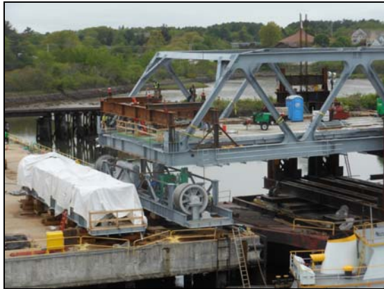
Figure 19 – Machine Room prior to installation, Jacking Grillage installed on Lift Span
