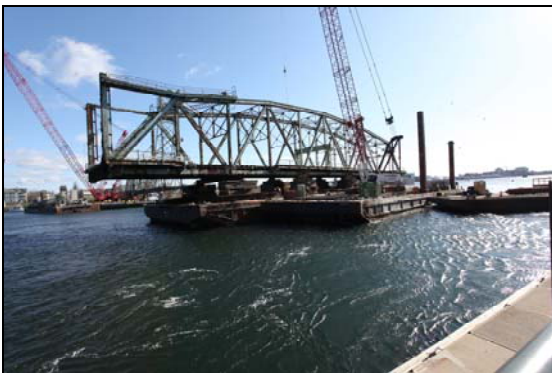
Figure 11 – Fixed Span removed and supported on barge
