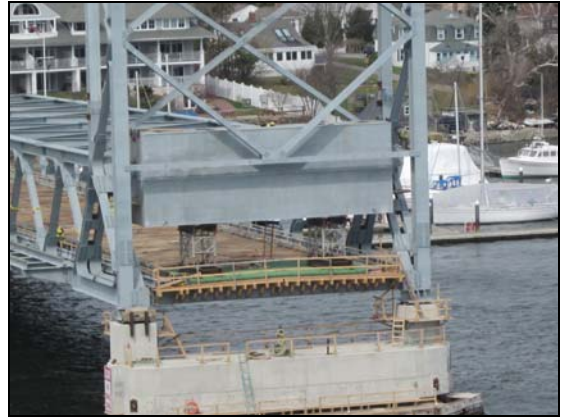
Figure 29 – New CTWT constructed on installed fixed span
