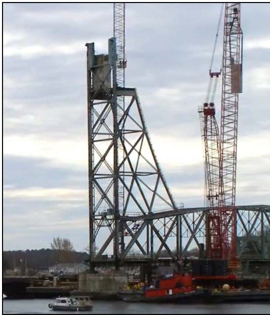
Figure 13 – Existing CTWT removal
