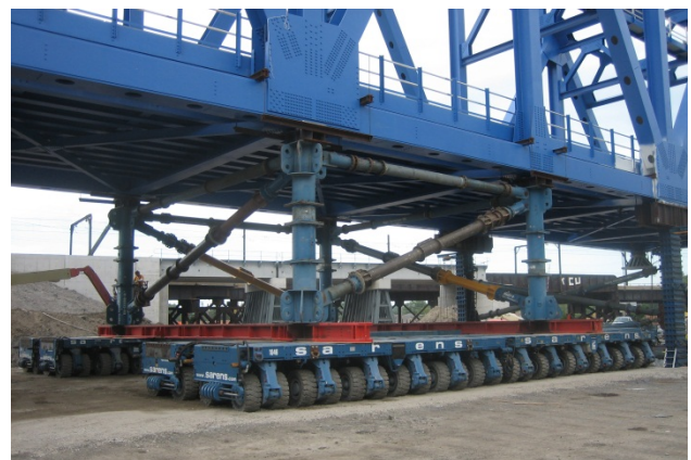
FIGURE 18 – (2) 24-Axle SPMT Groups and Support Structure Positioned Under Truss
