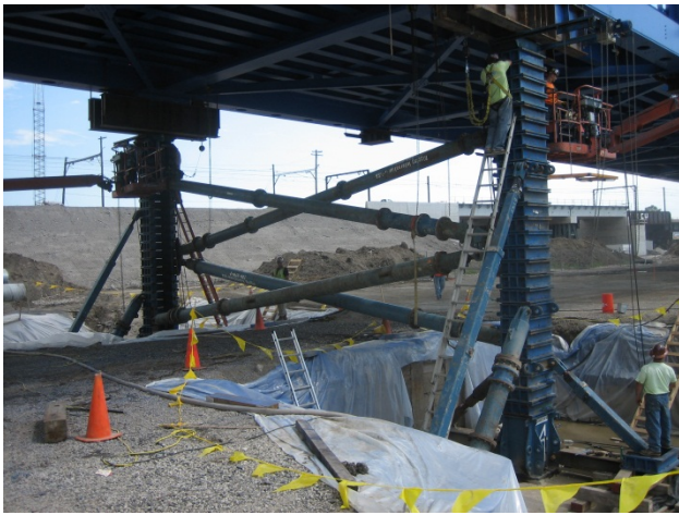
Figure 13 – Self-Climbing Tower With Bracing: Truss at Full-height of Lift
