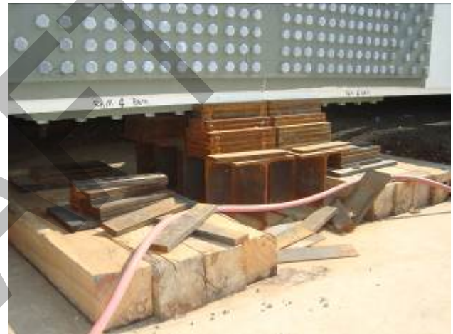
Figure 5 – Cribbing Supports for Truss Assembly
