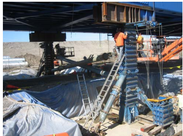
Figure 12 – Self-Climbing Tower With Bracing: Truss at Mid-Height of Lift
