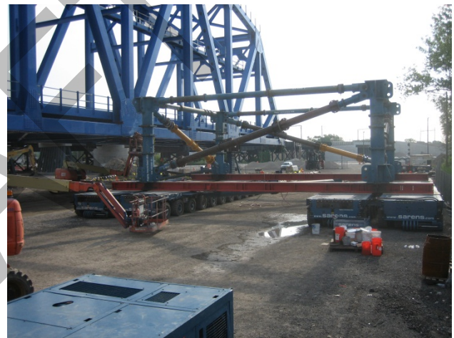
FIGURE 17 – Support Structure Built-Up on SPMTs – Prior to Move-In
