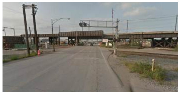
Figure 2 – At-Grade Roadway & Railroad Intersection Prior to Project Completion
