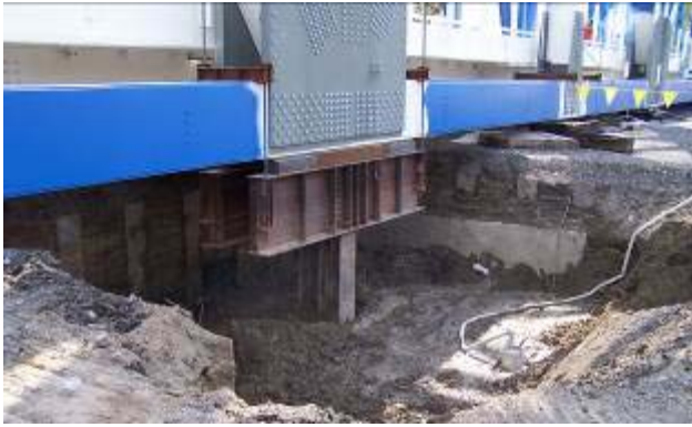
Figure 6 – Temporary Column Posts at Panel Points L2 & L10
