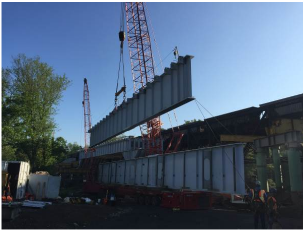
Figure 8 – Span 3 Unloading Off of SPMT
