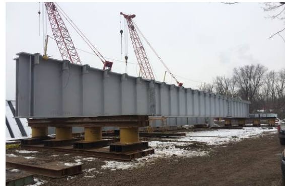
Figure 7 – Span 2 Girder Pre-Assembly
