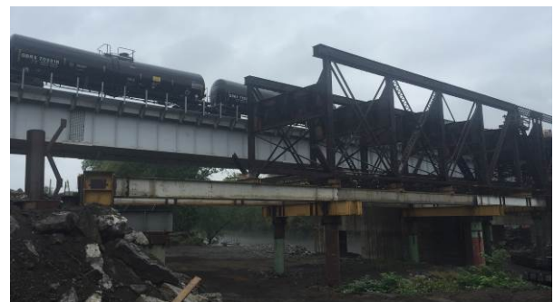
Figure 35 – Progressing Truss Demolition
