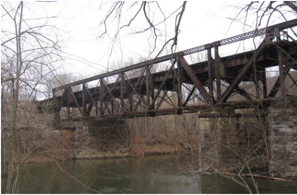
Figure 18 – Existing Truss Span
