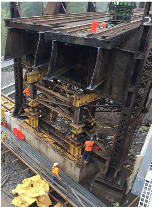
Figure 21 – Truss Lifting Frame Photo
