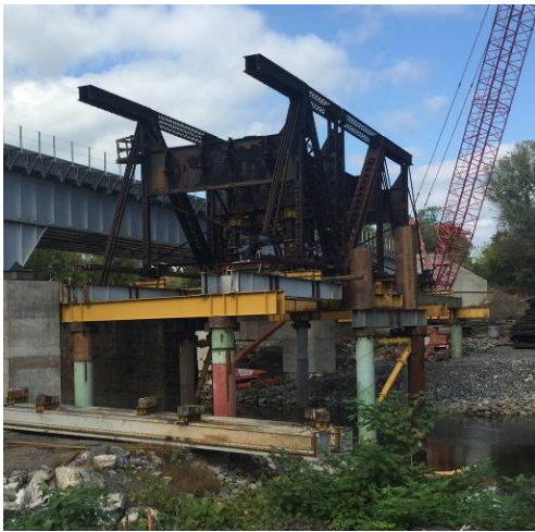
Figure 36 – Truss Demolition Nearly Complete
