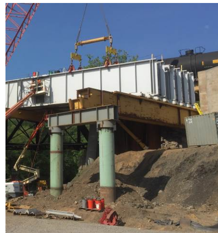
Figure 17 – Falsework Structures at Abutment
