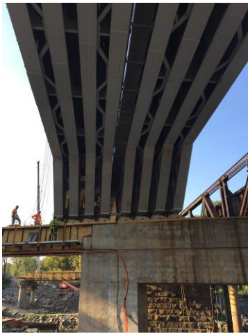
Figure 31 – Span Change-Out
