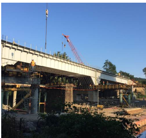
Figure 33 – Span Change-Out
