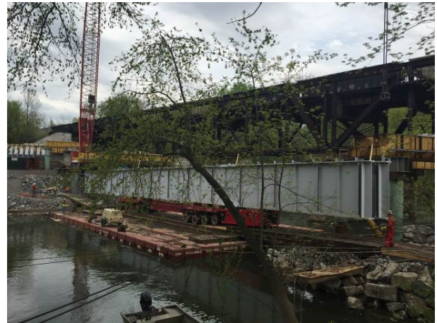
Figure 9 – Girder Transport on SPMT's Supported by Sectional Barges
