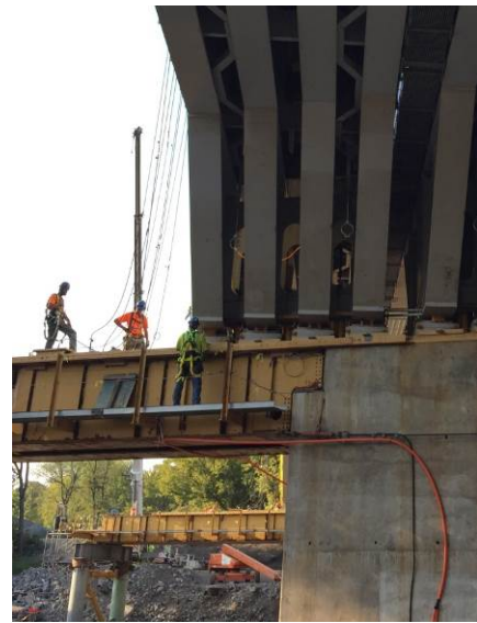
Figure 16 – Pier Modification for Support of Falsework Structures
