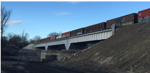
Figure 37 – Completed New Bridge
