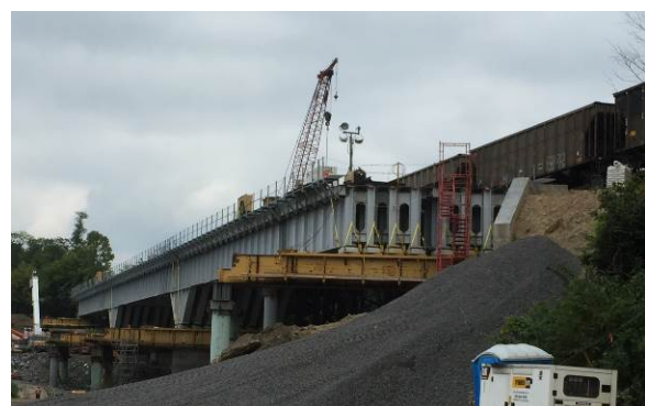
Figure 30 – New Steel Ready for Change-Out
