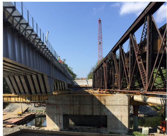
Figure 29 – Span Change-out
