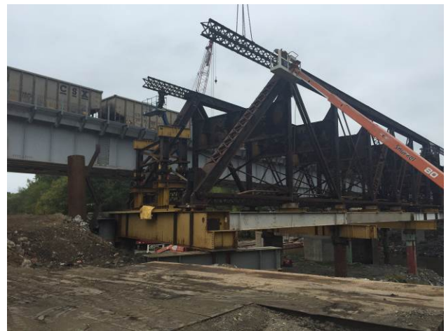
Figure 34 – Beginning Truss Demolition
