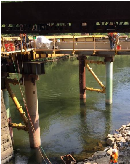
Figure 25 – Temporary Structure for Sliding Existing Truss Slide-Out
