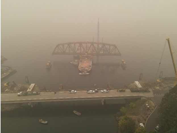
Figure 10 - New Truss Float In
