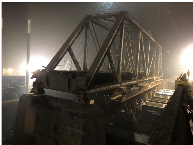
Figure 8 - Existing Truss Removal
