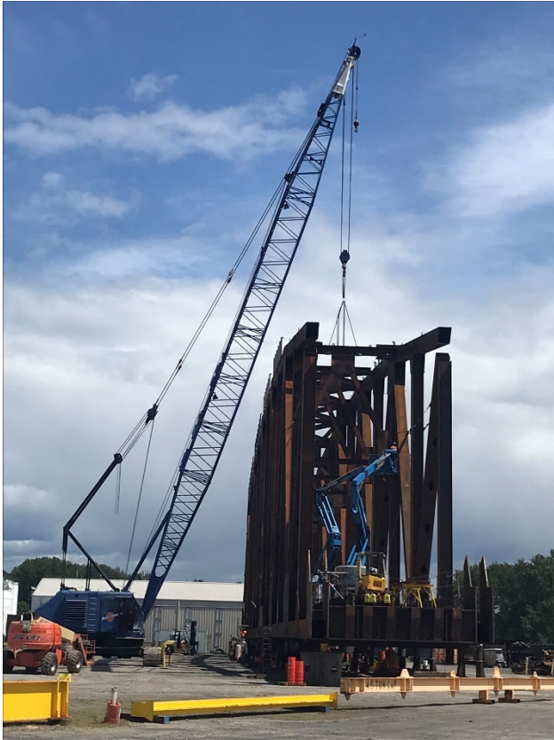
Figure 3 - Truss Assembly
