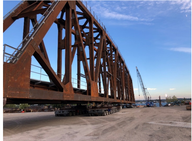
Figure 4 - Truss Roll On
