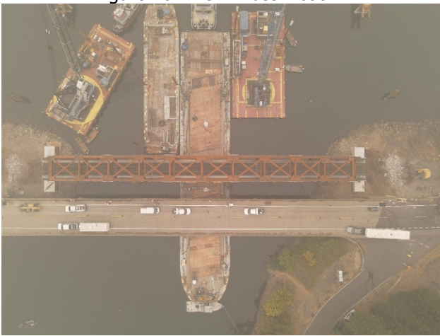
Figure 11 - New Truss Float In
