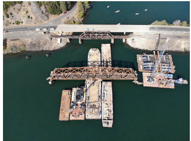
Figure 7- Float In Configuration
