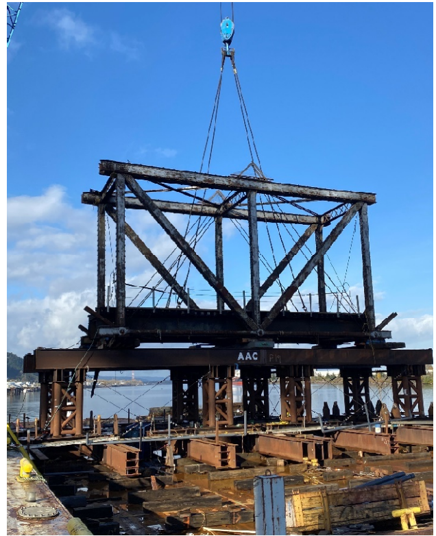
Figure 12 - Existing Truss Demolition
