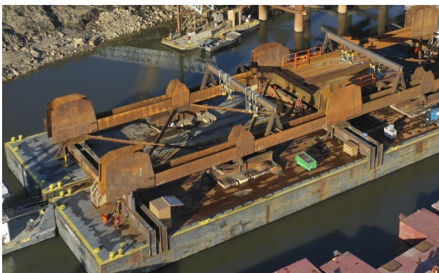
Figure 10 - Barge Grillage used for Truss Erection
