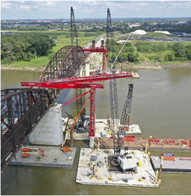
Figure 17 - Installation of Mammoet Gantry Beams. Downstream Falsework Temporarily Braced
