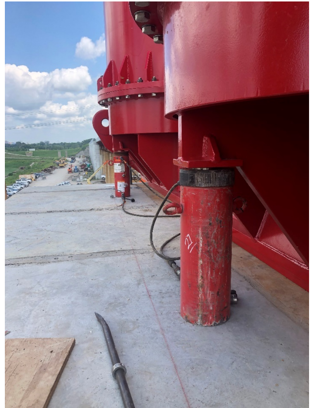
Figure 18 - Jacks used to help level upstream pier side columns.
