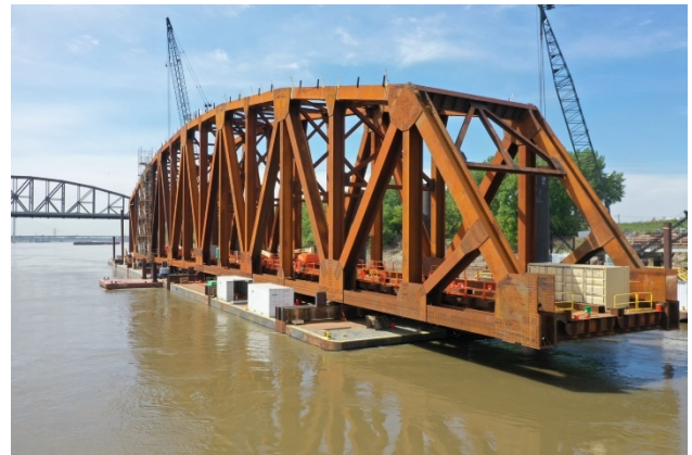
Figure 20 - New Truss Completed on Assembly / Float-in Barges – 2.5-ft of Freeboard Remaining
