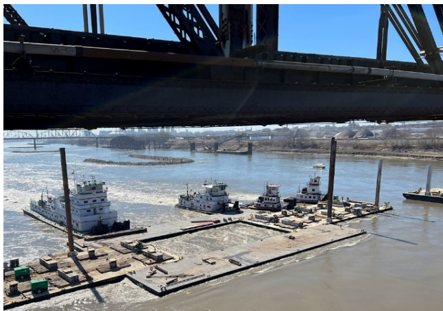
Figure 22 - Float-Out Barges Ballasted Down for Test Push with Tugboats
