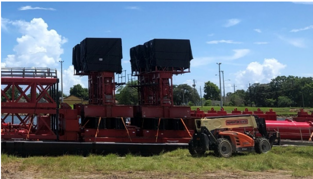
Figure 16 - Strandjack assembly with protective tarps
