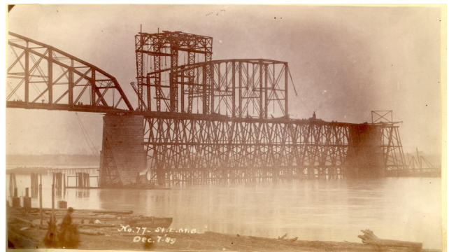
Figure 4 - Original Bridge Main Truss Span Construction
